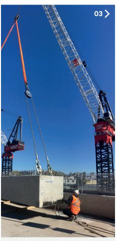
Using just two cranes in fixed locations, our methodology catered to the challenge of lifting elements weighing up to 60 tonnes, including some 50-tonne weights at the extreme ends and anywhere within and across the 200-metre station box.
