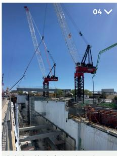
A critical consideration for the project was how to decongest the site. With cranes able to reach across the station box, we were able to facilitate a more efficient delivery unload and install process to lift pre-cast beams weighing up to 60 tonnes.
