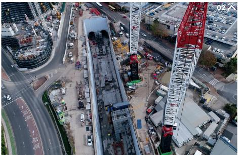
A birds-eye view of the congested site showing the position of the M1680D (foreground) and M2480D (background) in relation to the station box. Designed to meet the geotechnical considerations of the site, the position of the crane foundations adjacent to the station box allowed the cranes to carry out lifts on both sides of the construction area.
